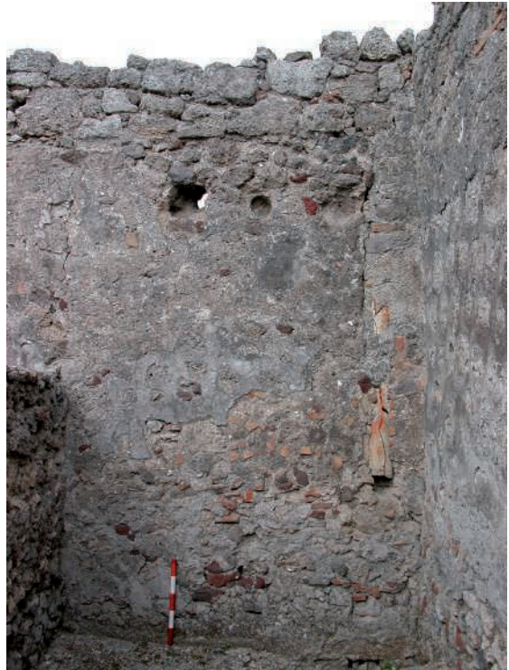
Fig. 7. Room 23 east wall showing immured downpipe from upper storey latrine.
