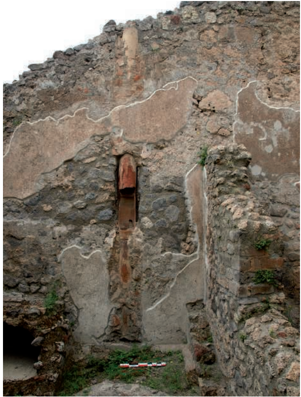
Fig. 2. North wall of kitchen (14), showing remains of downpipe from first floor latrine.
