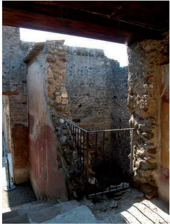
Fig. 5. North end of west side of room 19. Angle of plaster on north wall of staircase 17 indicates position of staircase described by Falkener.
