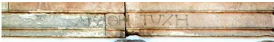
Ill. 4. The architrave of the Palazzo Castani in Milan.
