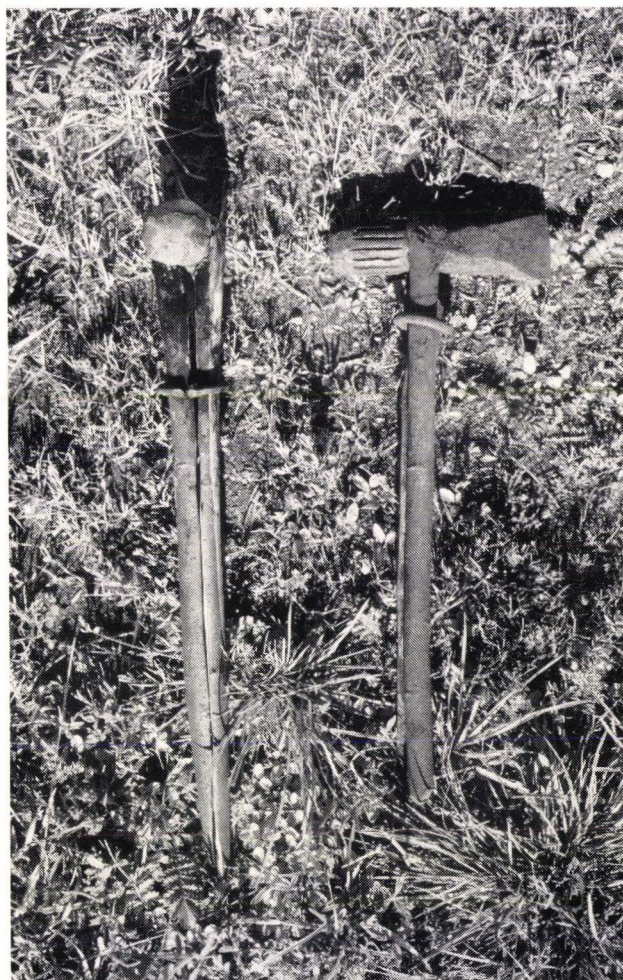
Fig. 5. Cutting irons from the smithy of Oiva Rännilä of Kuhmoinen. Willow withes are affixed to the irons. Photo Seppo Rintala 1985.
