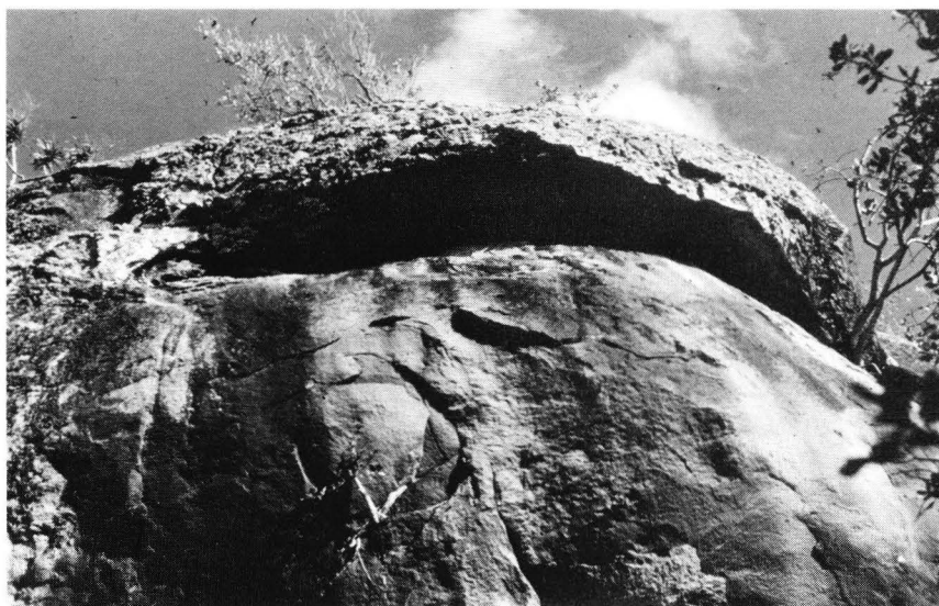
Fig. 5. Typical exfoliation of the basement rock (above KFR-A5).
