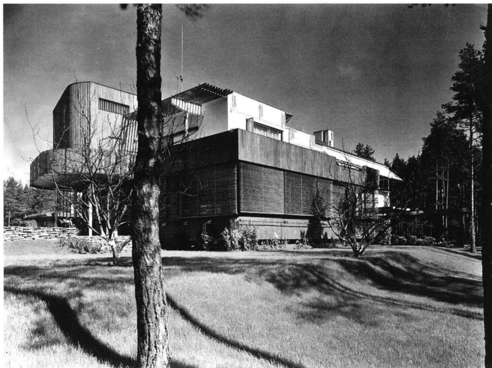
112. Villa Mairea at Noormarkku was built in 1938-1939. Alvar and Aino Aalto. SRM.
