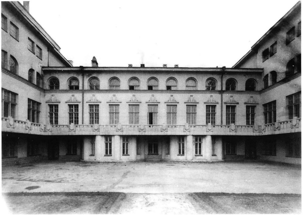
67. The original courtyard wing of the Estonia Theatre in 1913. Photograph by Parikas, ETM.
