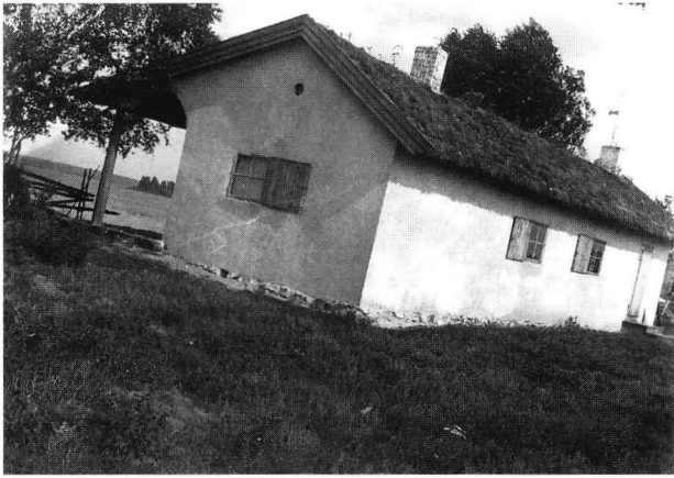
139. Villa Flora after completion. Photograph by Aino Marsio-Aalto. AAA.
