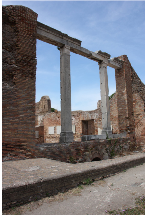
Figure 9. Terme del Foro. The view from the palaestra to the tepidarium 18: two rows of holes can be seen in the columns, used to fasten the wooden window-frames of the large windows opening towards the south. Photo: Arja Karivieri.
