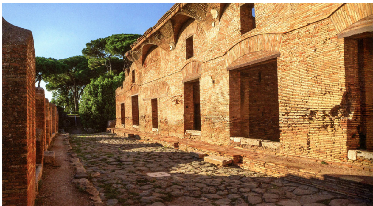
Figure 1. The shop entrances of the Casa di Diana opening onto the Via dei Balconi. Photo: Saana Säilynoja, Vapriikki Photo Archive.
