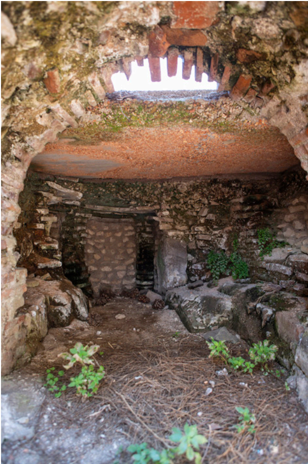
Figure 4. Entrance to a furnace beneath the raised floor in the Terme del Foro. Photo: Saana Säilynoja, Vapriikki Photo Archive.
