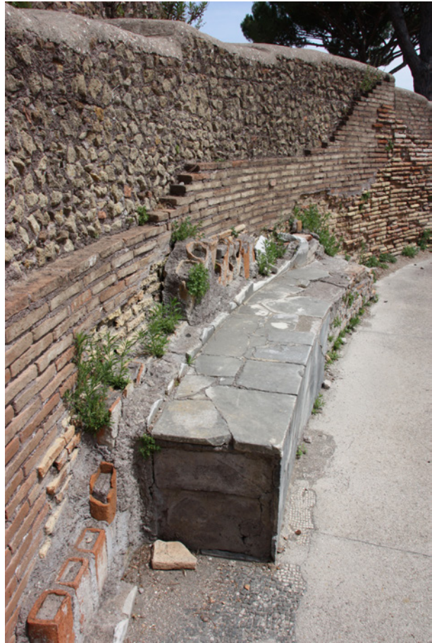
Figure 5. Terme del Foro. A row of the tile flues enabling hot air to circulate to the upper parts of the room can be seen behind the bench. Photo: Arja Karivieri.
