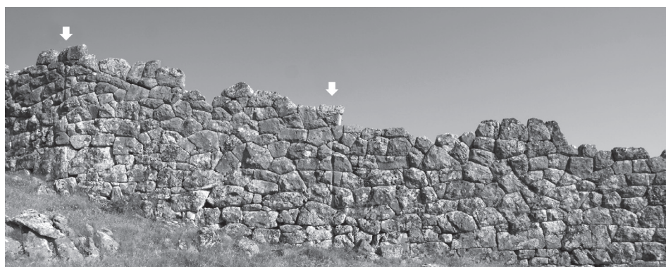
Fig. 18. The masonry styles after the bend. Note how, in the center of the photo, the masonry of the upper part stretches almost down to ground level. The arrows indicate the presence of two of the three vertical grooves in this curtain. View towards the south.
