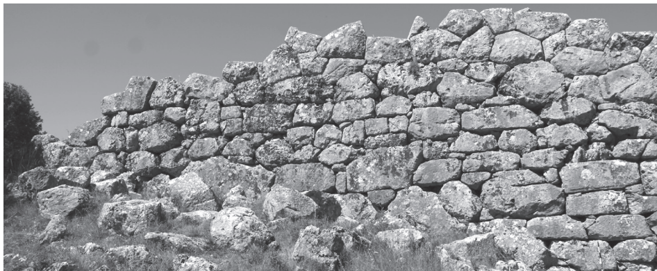
Fig. 11. The masonry in the southern end of the eastern curtain, on the left, is coarser than the one found in the following sectors. View towards the west.
