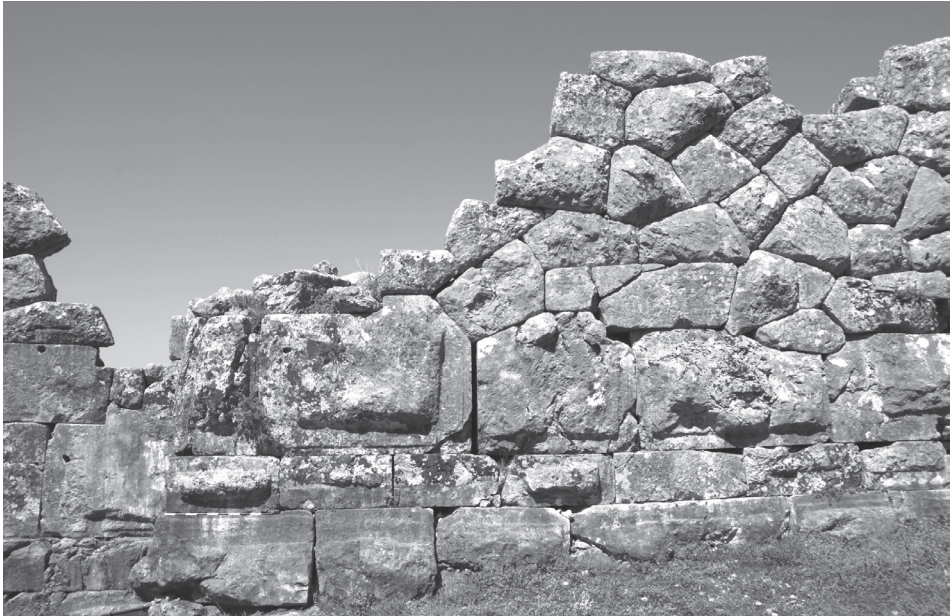
Fig. 16. The masonry used in the lower section of wall between the jog and the tower is very different. Large blocks have wide tooled margins, while the hammered central panel bulges very strongly. The footing course has a wide, smooth band along the upper edges of the blocks.
