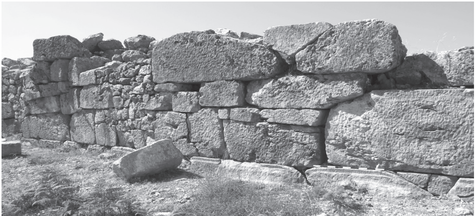
Fig. 23. The curtain has a peculiar footing course, seen below the stick. All the blocks in the footing have a smooth band on their upper sides. View towards the southwest.
