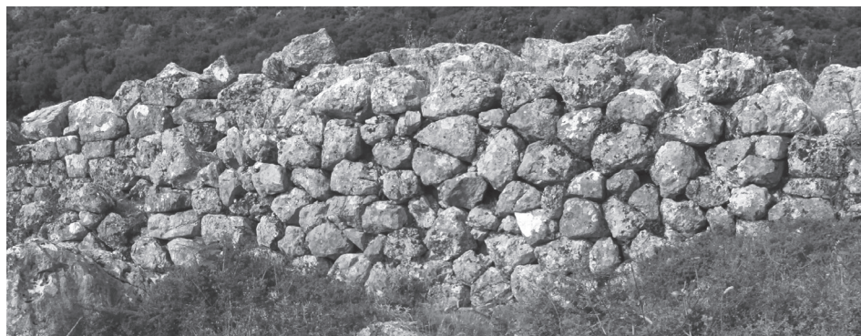
Fig. 14. The inside face of the bastion. Note how extremely rough the masonry and the joints are, when compared to the adjacent curtain, visible on the left and in Fig. 13.
