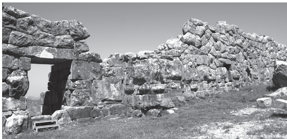
Fig. 15. The outer face of the northeastern curtain. The huge block mentioned in the text sits on top of the foundation, next to the jog. Note how different the masonry is in this area.
