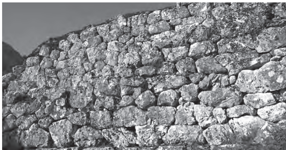
Fig. 13. The inner face of the same curtain. Note the protruding foundation with level top at the bottom, the rough appearance of the following section and the slightly more accurate finish in the thinner upper part.
