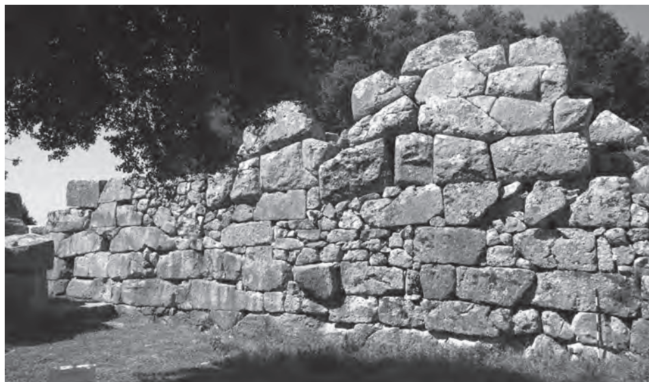
Fig. 21. The best preserved stretch of the northern curtain, showing the masonry styles used. On the left, the Northeastern Gate is just visible. The restorers have filled the holes in the wall with small stones. View towards the southwest.
