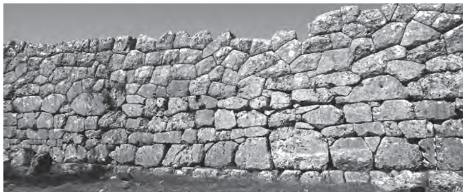
Fig. 12. The masonry in the outer face of the eastern curtain. Note at the bottom the shallow footing course with a level top, the following large, tooled-faced masonry, above which is the neat, quarry- or hammer-faced polygonal masonry. The frequency of triangular plugs in the lower section is also noteworthy.
