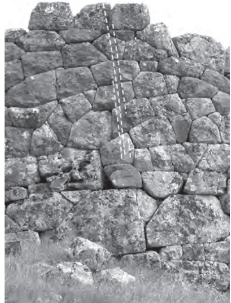
Fig. 19. The crooked groove cut into the bend of the northeastern curtain. The cuts are indicated by the dashed line.
